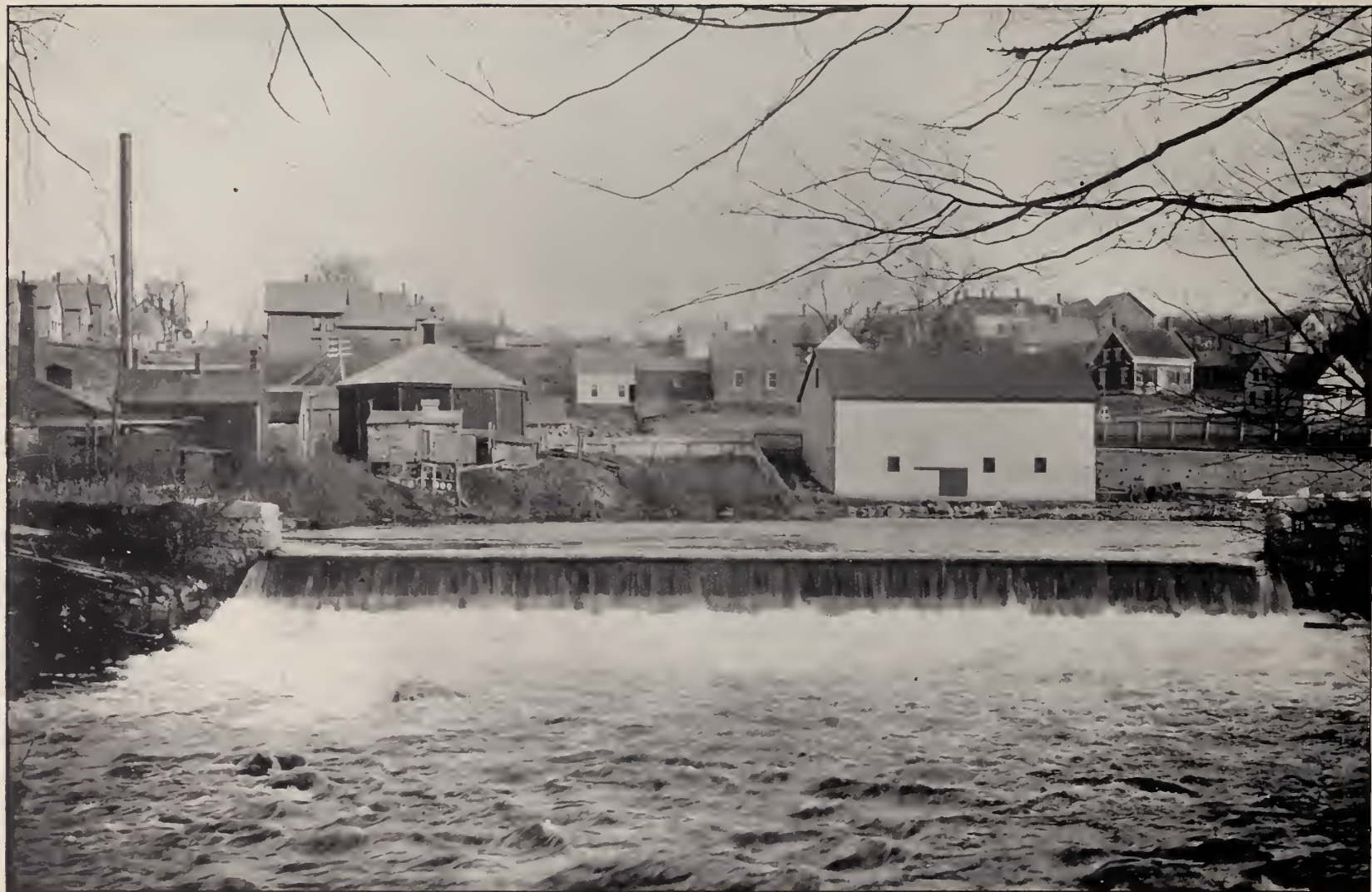
DAM NO. 3, OWNED BY THE GARDINER REAL ESTATE ASSOCIATION.—FALL 16.50 FEET. See Page 99.
